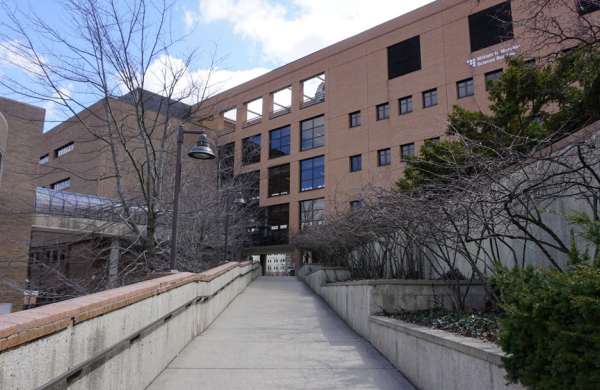
19. University of Michigan - Flint / Address: 303 Kearsley Street Architect: Various
