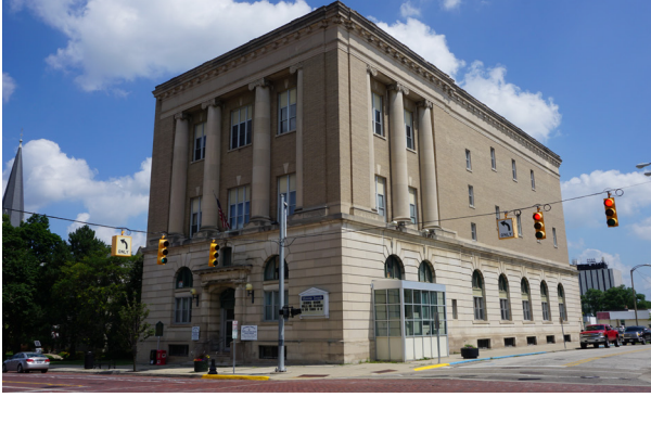
21. Flint Masonic Temple Address: 755 Saginaw Street Architect: H.B. Clement, 1911
